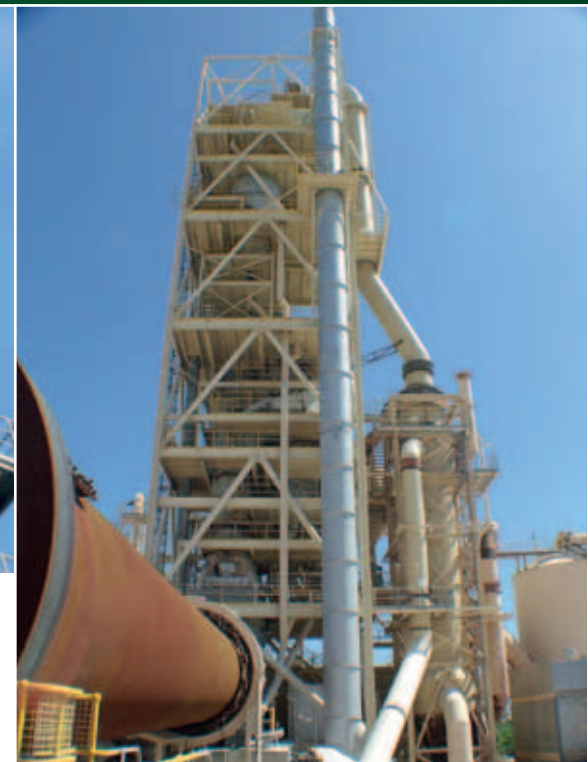
Lime production plant in Australia. The material – dune sand – is processed in a shaft-type flash dryer, cyclone preheater and rotary kiln before being cooled in a flash cooler.
