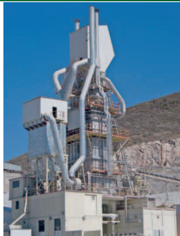
Maerz parallel-flow regenerative lime shaft kiln in Mexico.
