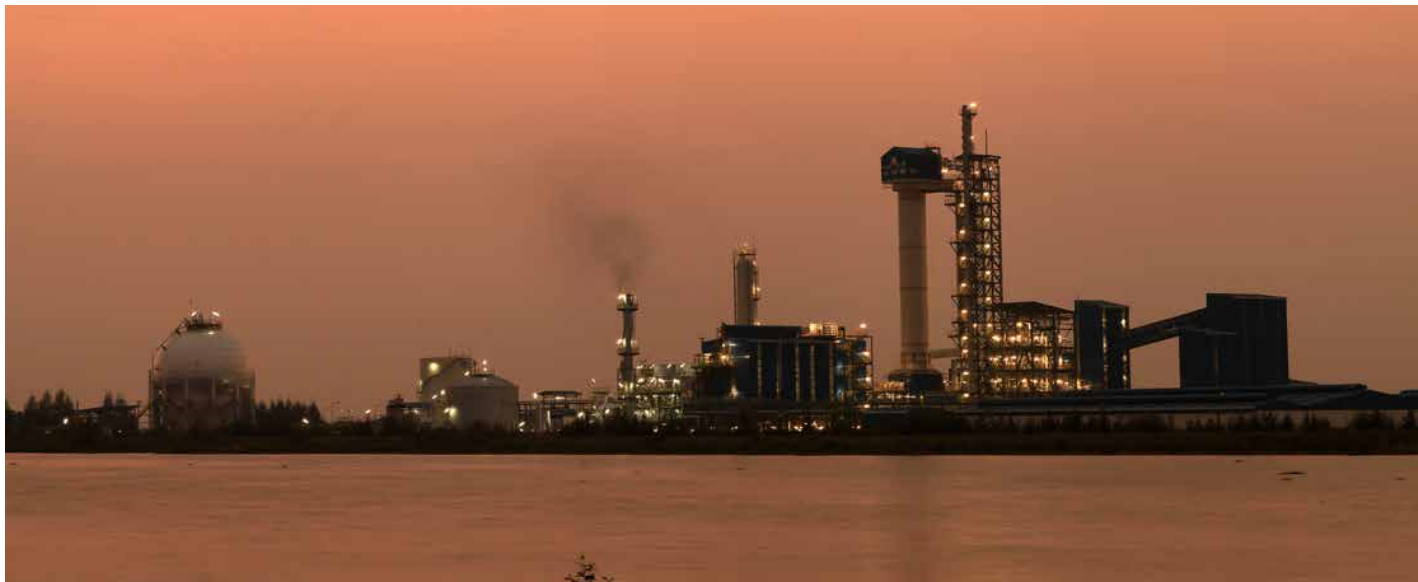
Ammonium nitrate prilling complex for VINACOMIN-Mining Chemical Industry Holding Corp. Ltd., Vietnam. Capacity: 625 t/day AN prills (technical grade)
