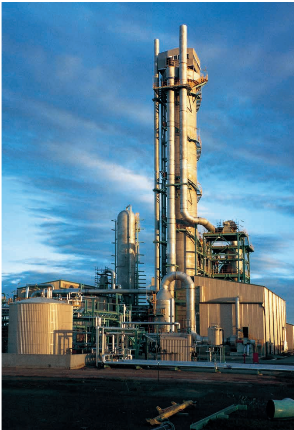
Ammonium nitrate prilling unit for Queensland Nitrates Pty Ltd., Australia. Capacity: 400 t/day AN prills (technical grade)
