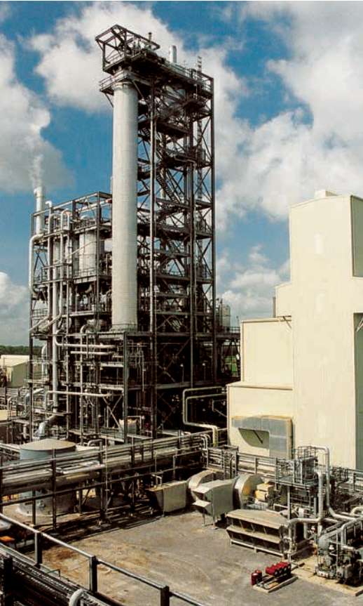
Fertilizer complex for CF Industries Inc. in Louisiana, USA including a 2,000 t/day urea plant, a 870 t/day nitric acid plant, a 1,105 t/day AN plant and a 2,450 t/day UAN solution plant.
