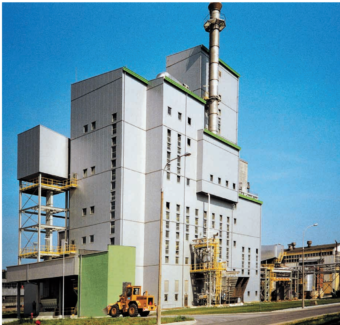
Pugmill granulation unit for ANWIL S.A. in Wloclawek, Poland. Capacities: 1,200 t/day AN granules and 1,500 t/day CAN granules
