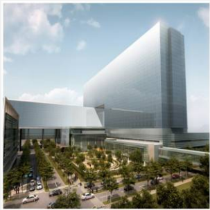
New Parkland Hospital Dallas, USA
