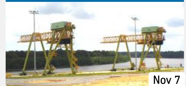
1 st CSA Slabs Arriving in Mobile
