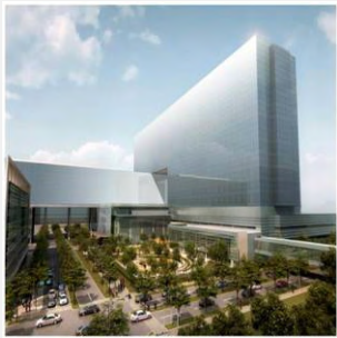
New Parkland Hospital Dallas, USA
