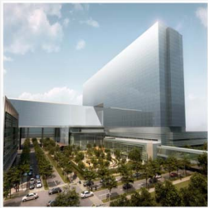
New Parkland Hospital Dallas, USA
