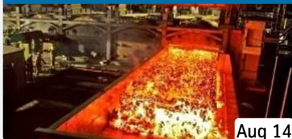
1 st Push Coke Plant
