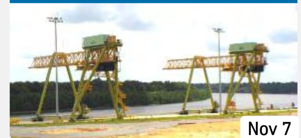
1 st CSA Slabs Arriving in Mobile
