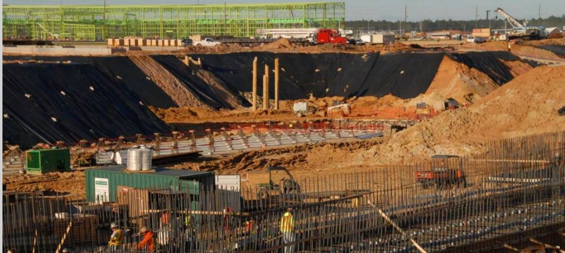
Cold-rolling mill: foundation work
