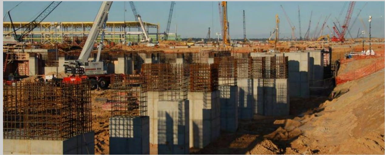
Coating lines: foundation work
