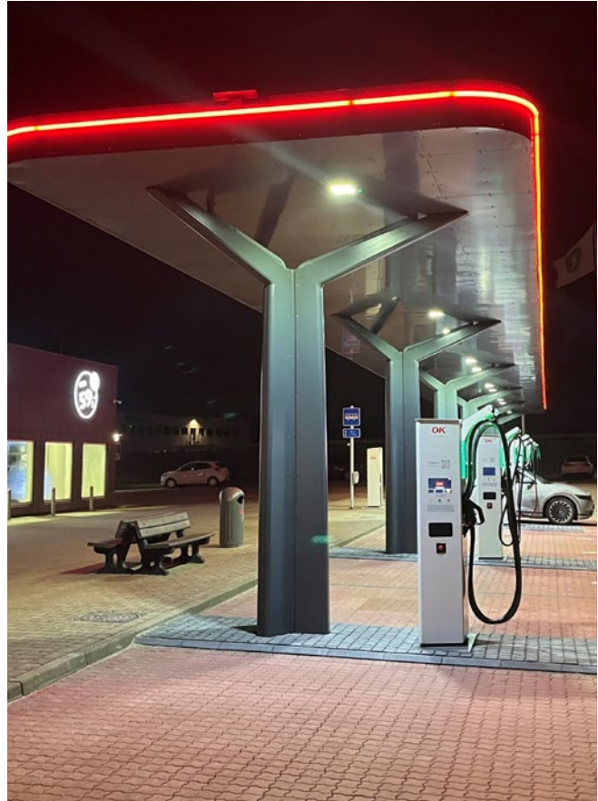
Carports and charging stations, Denmark
