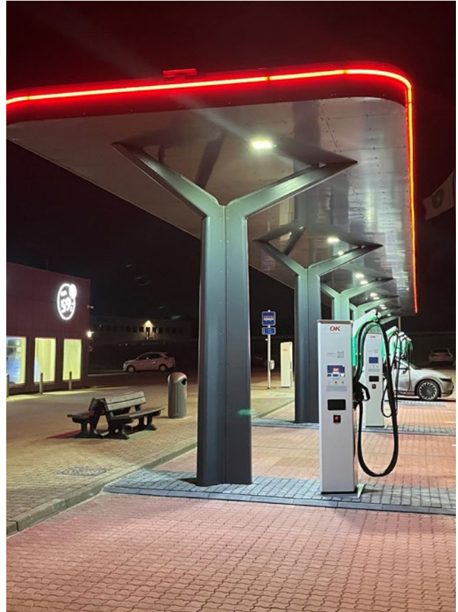
Carports and charging stations, Denmark
