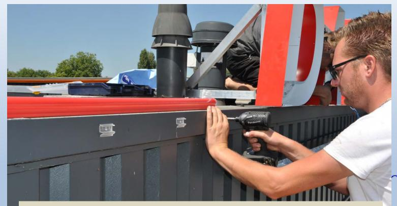
Per 2370 section use 6 sliding clips, 3 left and 3 right of the fixed clip. Not more than 400 mm apart.
