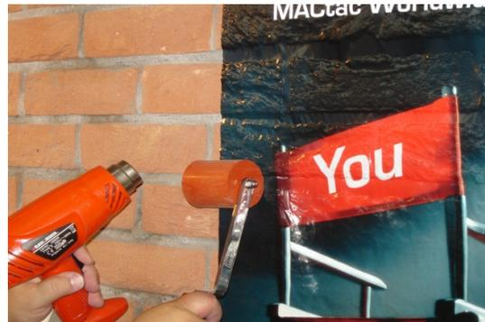
\* After you have established or are satisfied with the definite position of the graphic, apply firm pressure to the printed image, using a semi-hard roller (**the Wheelie**). The structure of the bricks will show up through the film.
