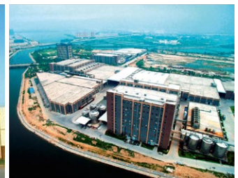
PA 6 two-stage polymerization 54,000 t/year (one line) with DRP® DSM Chinalon, Jiangyin, China (top left)
