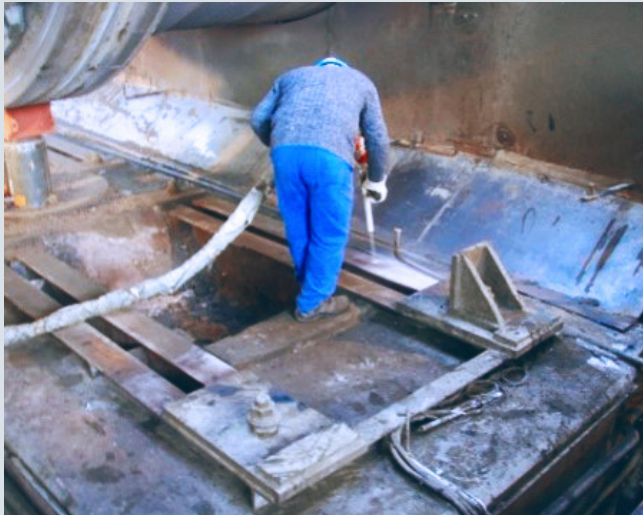
Removal of the old roller units and cleaning of the existing baseplate. No work is required on the baseplate or the kiln foundation.
