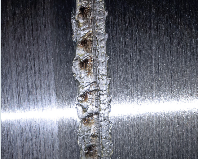
Damage to a mill slide ring
