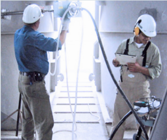
Dust measurement in the preheater
