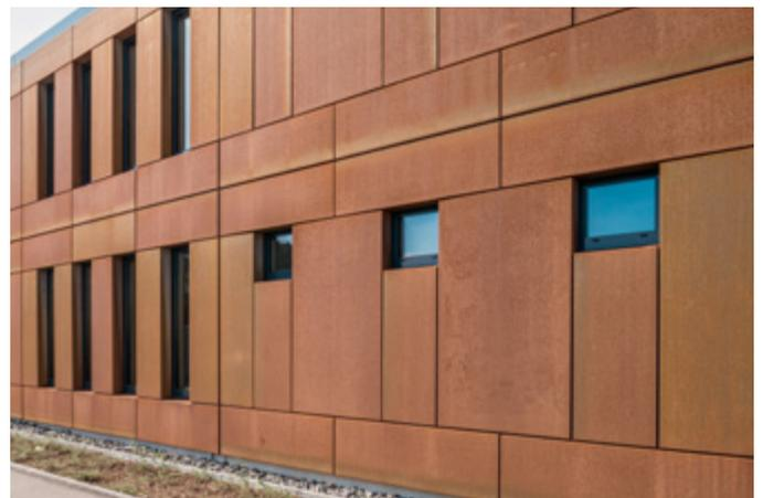
Weathering steel in use – Façades panels made of patinax®.
