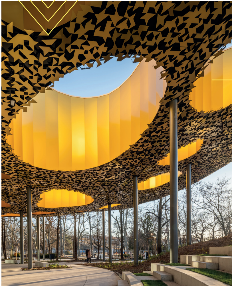
House of Music, Hongrie Sou Fujimoto Architects ALUCOBOND® PLUS spectra Desert Gold © György Palkó
