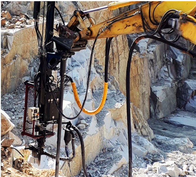
HB5 drilling in a granite quarry
