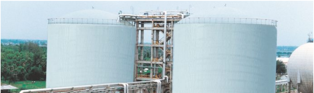
Cryogenic Ammonia Storage Tanks with associated facilities
